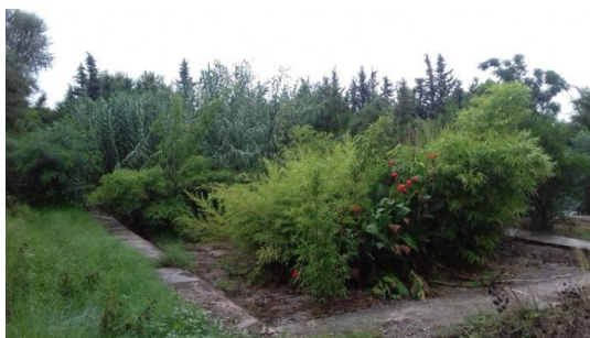
Fig 1 : Treatment plant for Jougar village
